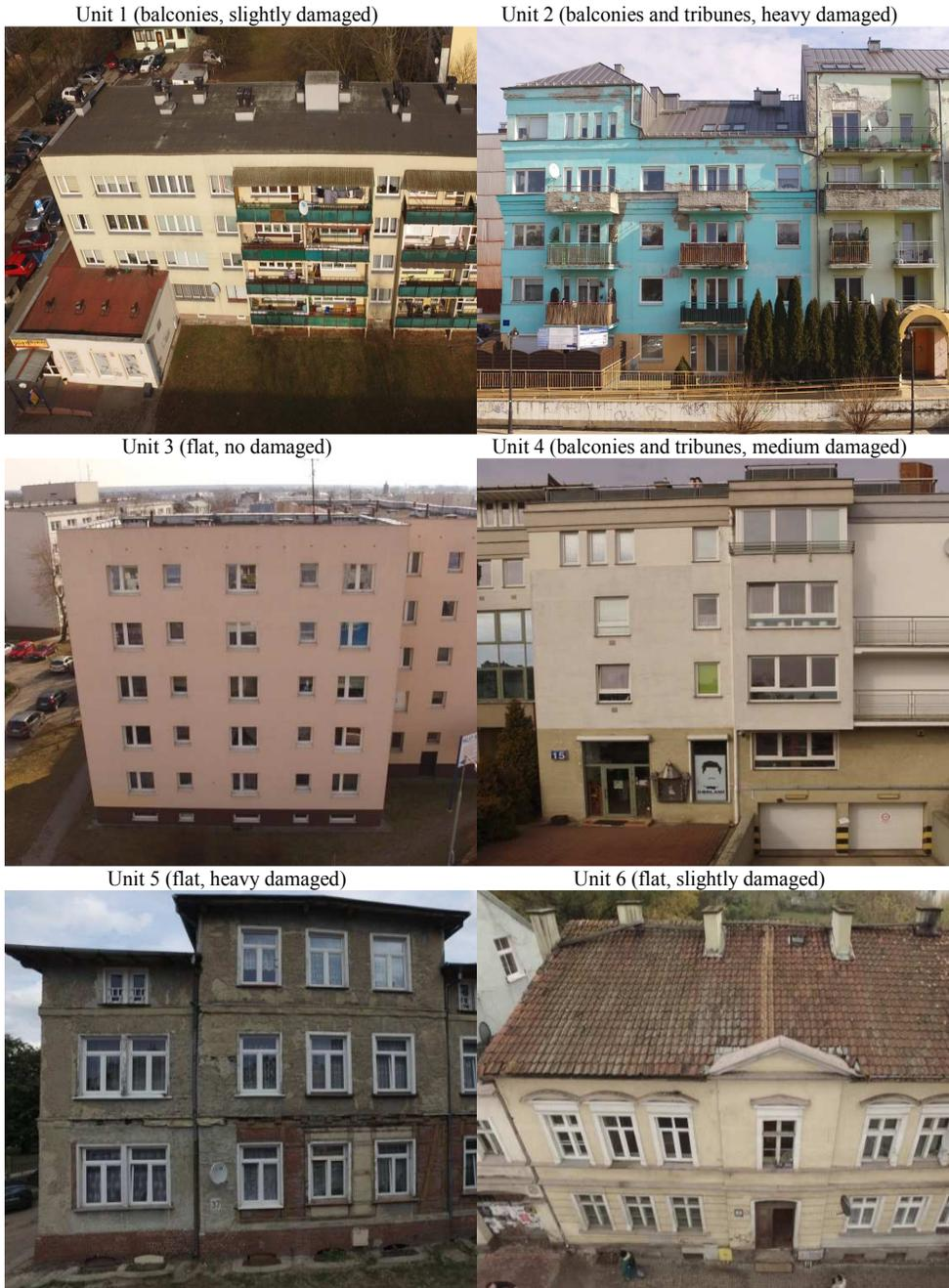
**Fig. 2.2.** General views of the facades in the sample. In parentheses (morphology, deterioration level)
